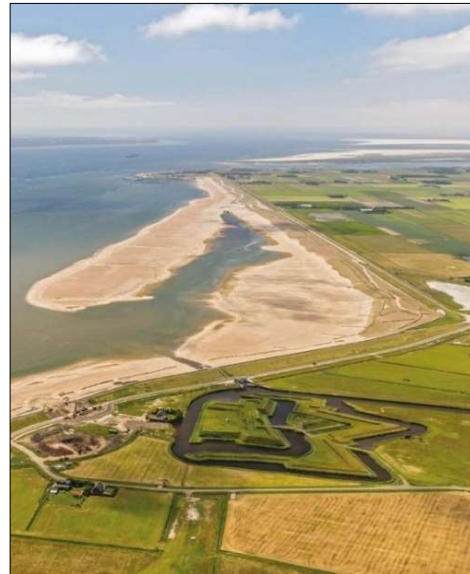
Prins Hendrik Zanddijk project in the Netherlands
